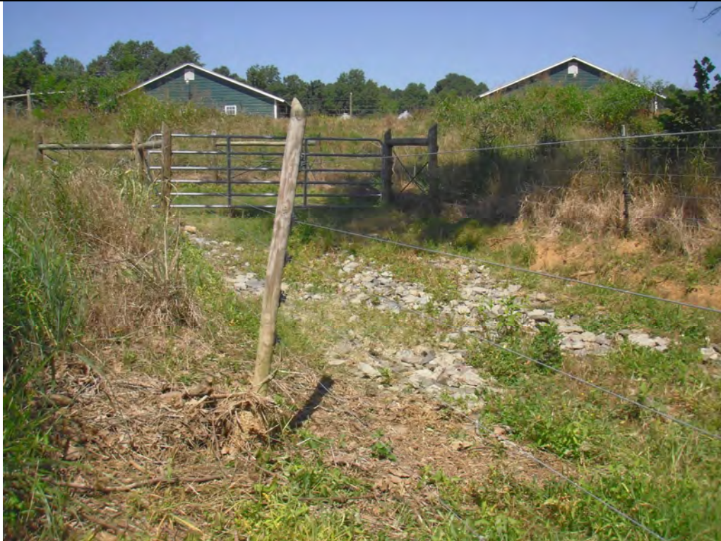
SP3: Rack line along ford crossing approximately above Design Bankfull elevation Taken On: 2010
