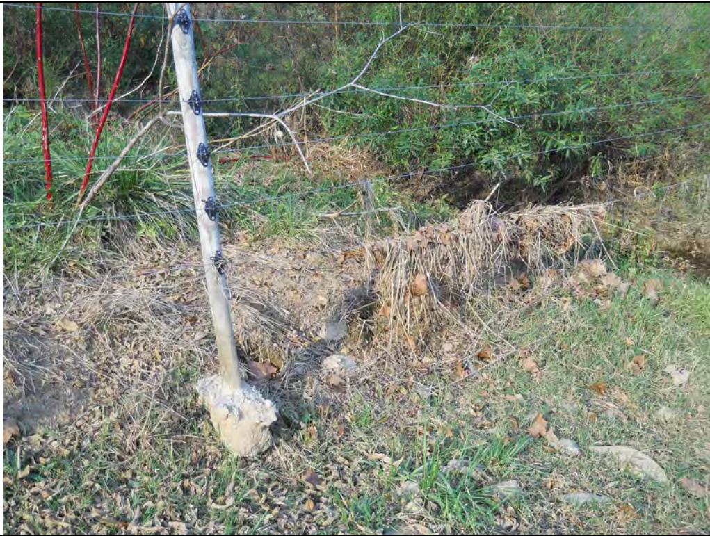
SP1: Fence damage at UTJC1 with rack line Taken On: 2010
