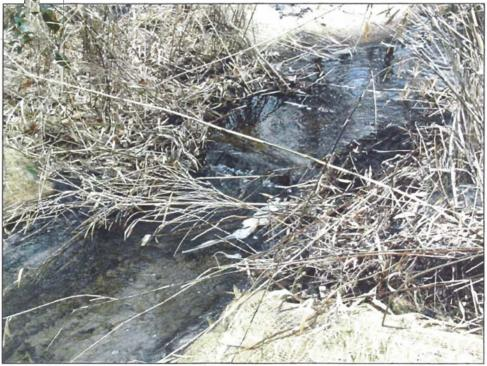
Photo **P4**. A completed log weir structure. The log weir is used to set the grade of the **streambed upstream** of the structure **and** keep the channel **from** downcutting. Log weirs also provide habitat features (Feb. 28,2003).
