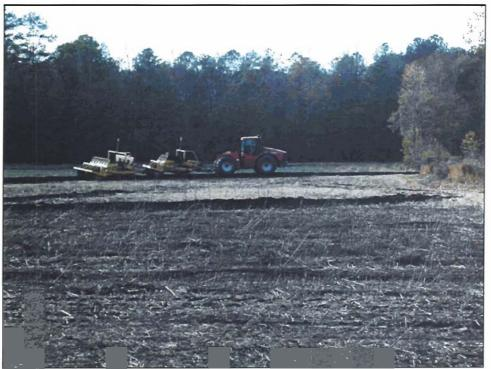
Photo C1. Minor grading of the site was performed to remove field crowns and provide fill material for ditches on the site (Nov. 22,2002).
