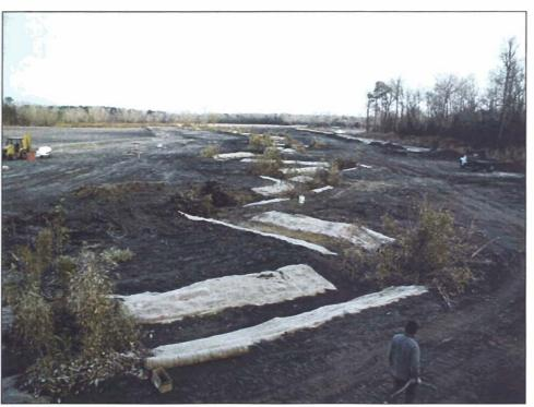
Photo C8. The last segment of new channel is completed at the upstream end of the project and ready to receive water (Jan. 16, 2003).
