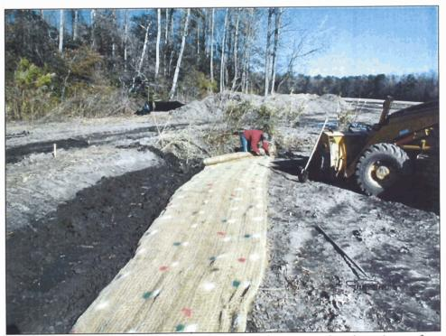
Photo C6. Installation of coir fiber matting along completed sections of new streambank (Dec.16, 2002).
