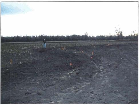
Photo C2. A section of channel excavated and ready for the installation of structures, transplants, and matting. The orange stakes mark the design top of banks (Dec. 2,2002).
