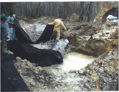
Photo C5. Construction of one of the cross-vane structures installed at the outlet end of the project. Cross-vanes control the bed elevation of the new stream and protect the stream from downcutting (Dec. 4, 2002).
