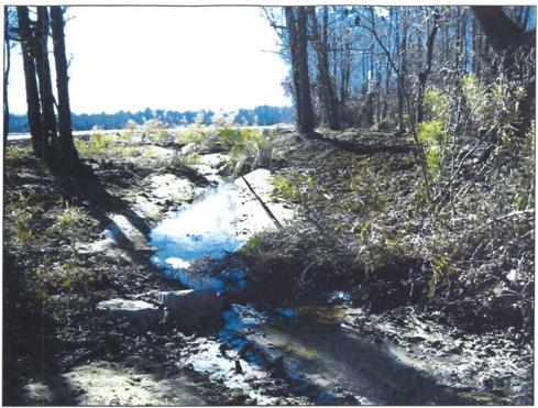
Photo P1. The downstream end of the **project where** the new **channel** connects with the existing channel **and** Mill Creek. Two cross-vane structures are visible in this picture(Jan. 28,2003).
