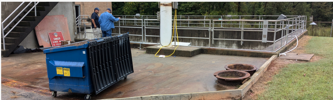
Figure 9. Member Facility Two Rivers Utilities
