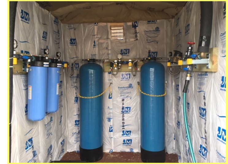
Whole-House Granular Activated Carbon system
