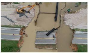
Figure 5J-5: The Little River washed out US- 401 in northeast Wake County
