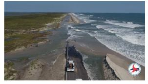
Figure 5J- 5: NC-12 on Ocracoke Island washed out after Hurricane Dorian
