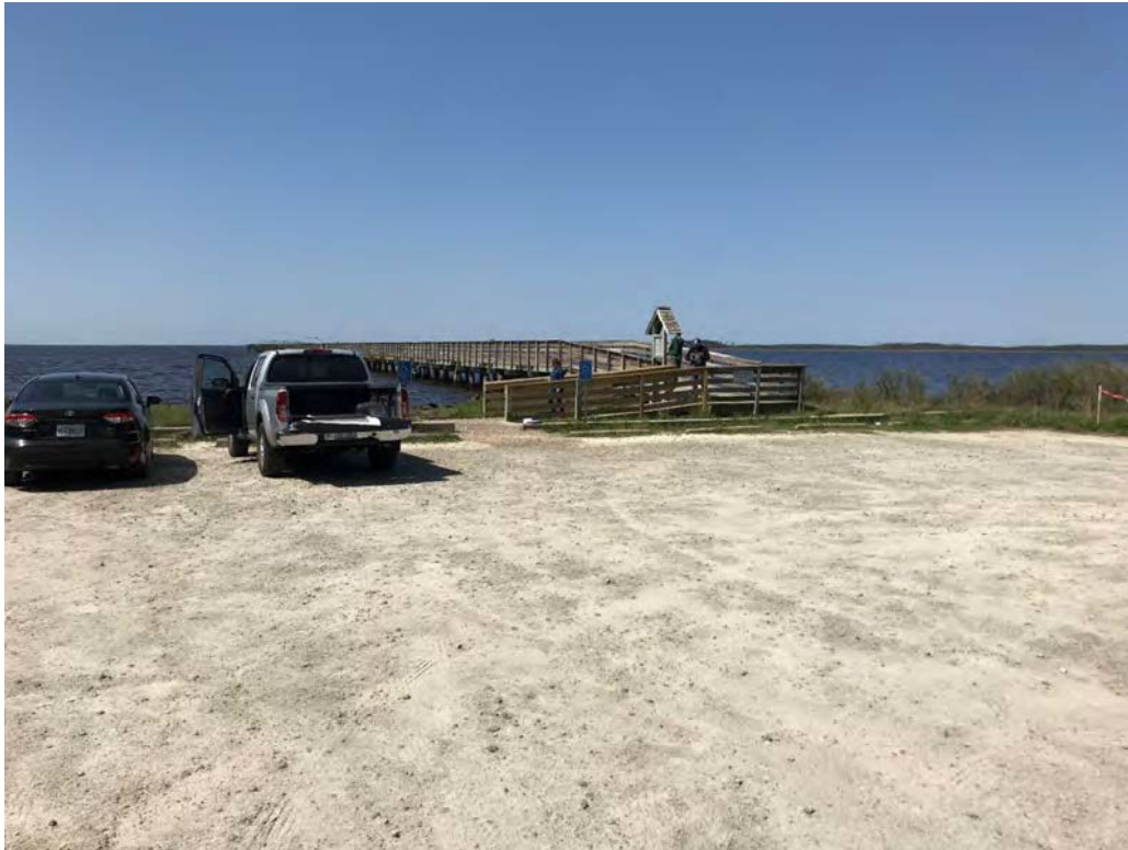
Figure 5: Looking west at current ramp to pier and current parking area.
