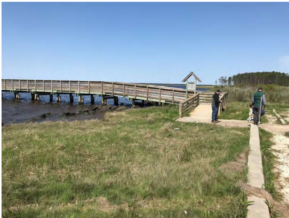
Figure 4: Looking NW at current ramp to access the pier.
