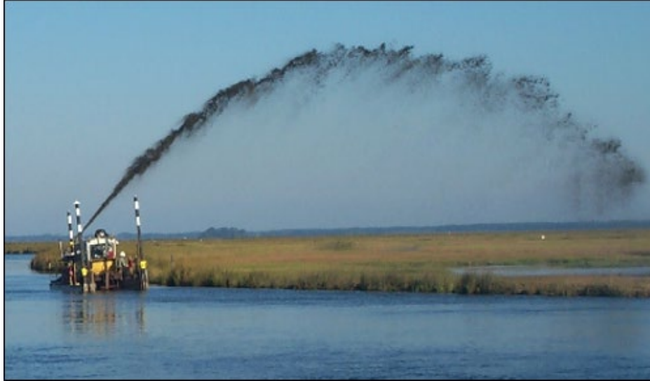
Fig. 2: Typical method used for thin layer placement (Image Source: U.S. Army Corps of Engineers)
