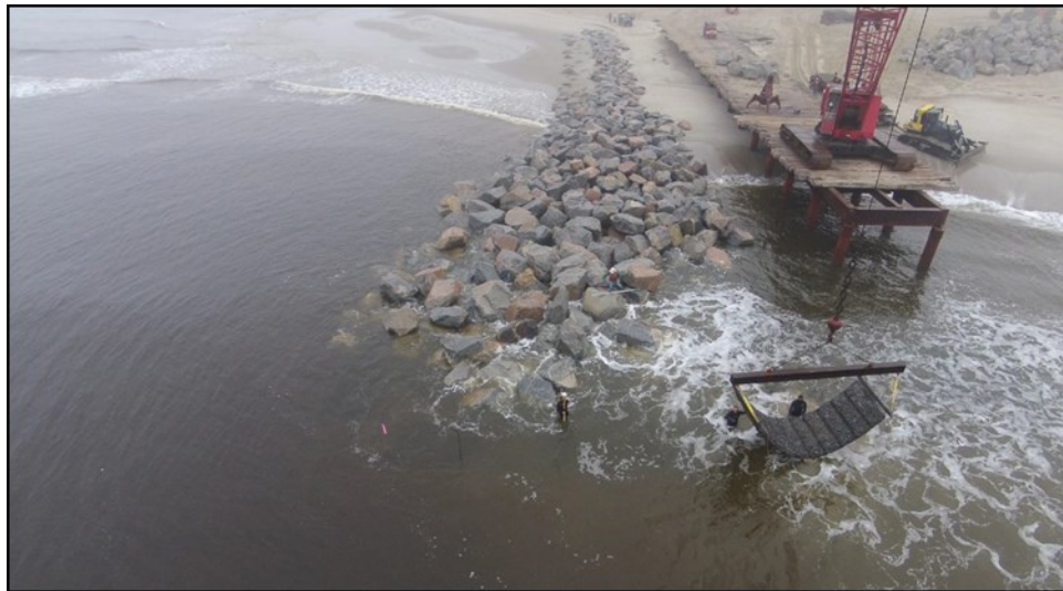
Figure 10. Terminal groin being installed at the Village of Bald Head Island in 2015. Photo: Village of Bald Head Island, 2015
