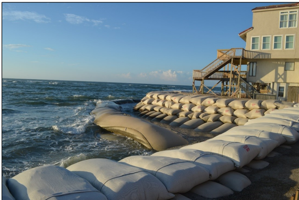
Figure 22. Sandbag structures at North Carolina's North Topsail Beach have been successful in providing short-term home protection from erosion at the expense of losing a sandy beach. Photo: NCDCM, 2015
