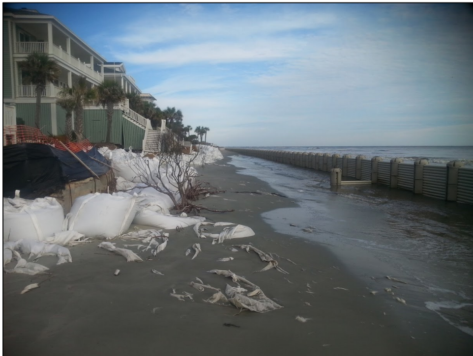
Figure 14. Experimental erosion control structure installed at land-ocean interface at Isle of Palms, S.C. with partially damaged sandbags behind the structure. Photo: NCDCM, 2015
