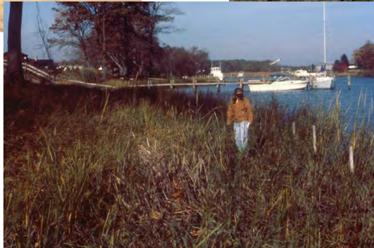
Stone Containment Structure
