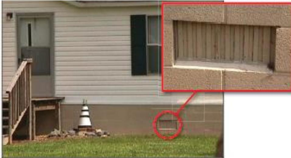
Figure 17: Standard air vent that is unacceptable as a flood opening because it is not disabled in the open position
