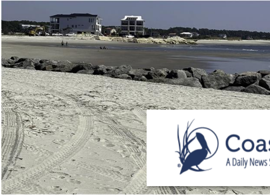
A view looking east of Ocean Isle Beach's terminal groin, where sandbags hold off beachfront erosion. Photo: Trista Talton
