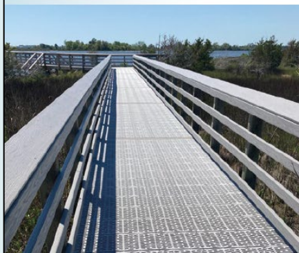
Examples of flow-through decking at the Morris Landing Clean Water Preserve
