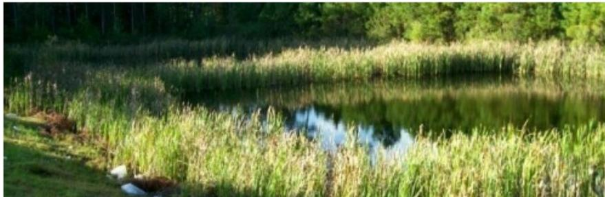
*Wet ponds improve stormwater quality by holding stormwater over a two to five day period. A wet pond includes a forebay, a permanent pool, and a temporary*
