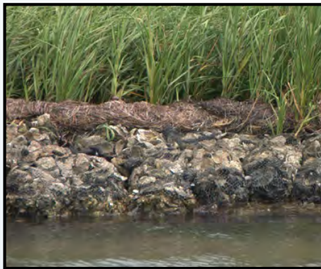
Example of Oyster Shell Bag Marsh Toe Revetment.
