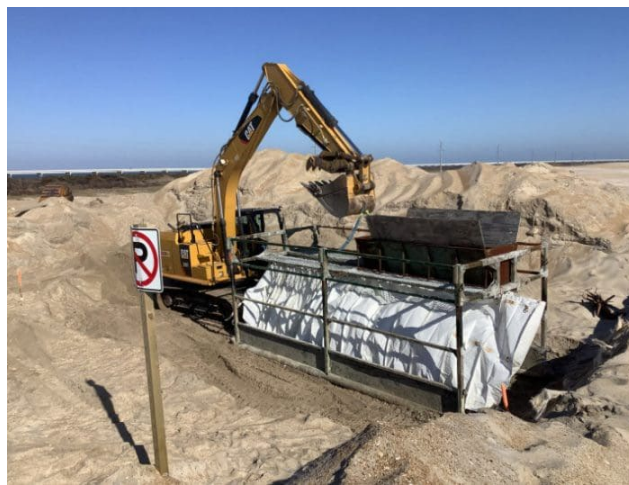
Figure 1. Alternative sandbag being installed at Pea Island. Photo: Division of Coastal Management
