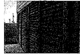
BREAKAWAY WALL FIXED LOUVERS
