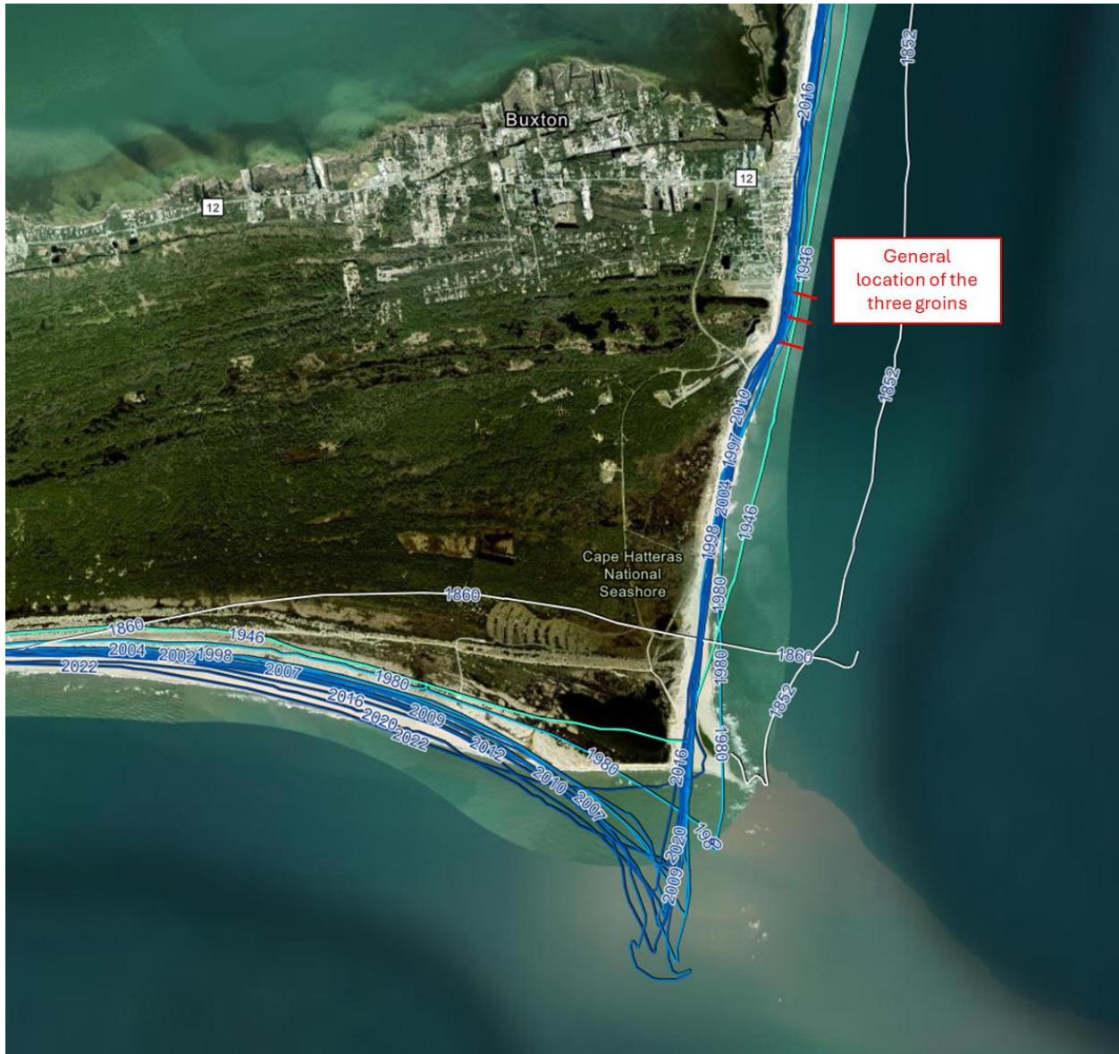
Figure 4. Generalized location of three shore-perpendicular rock and steel groins constructed by the U.S. Navy between 1969 and 1970 to protect former military infrastructure near the Cape Hatteras Lighthouse, NC. Shoreline positions from the NCDRCM database are overlaid on 2024 aerial imagery. The groins are not depicted to scale and are commonly referred to as the 1st, 2nd, and 3rd “jetty,” progressing from south to north.
