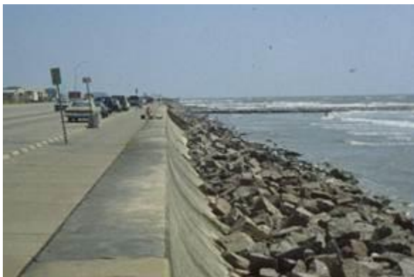
Figure 12. The Galveston Seawall.
