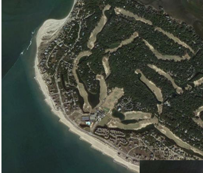
Aerial view of geotextile sand tubes, 2013
