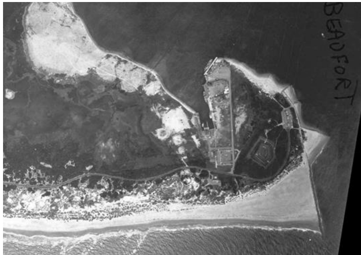
1971 photo, after terminal groin construction, USACE
