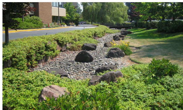
Landscaped retention ponds and swales collect and treat stormwater and can also function as parks or amenities.
