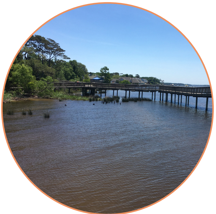
The town boardwalk provides a view of saltwater marsh wetlands and submerged aquatic habitat.
