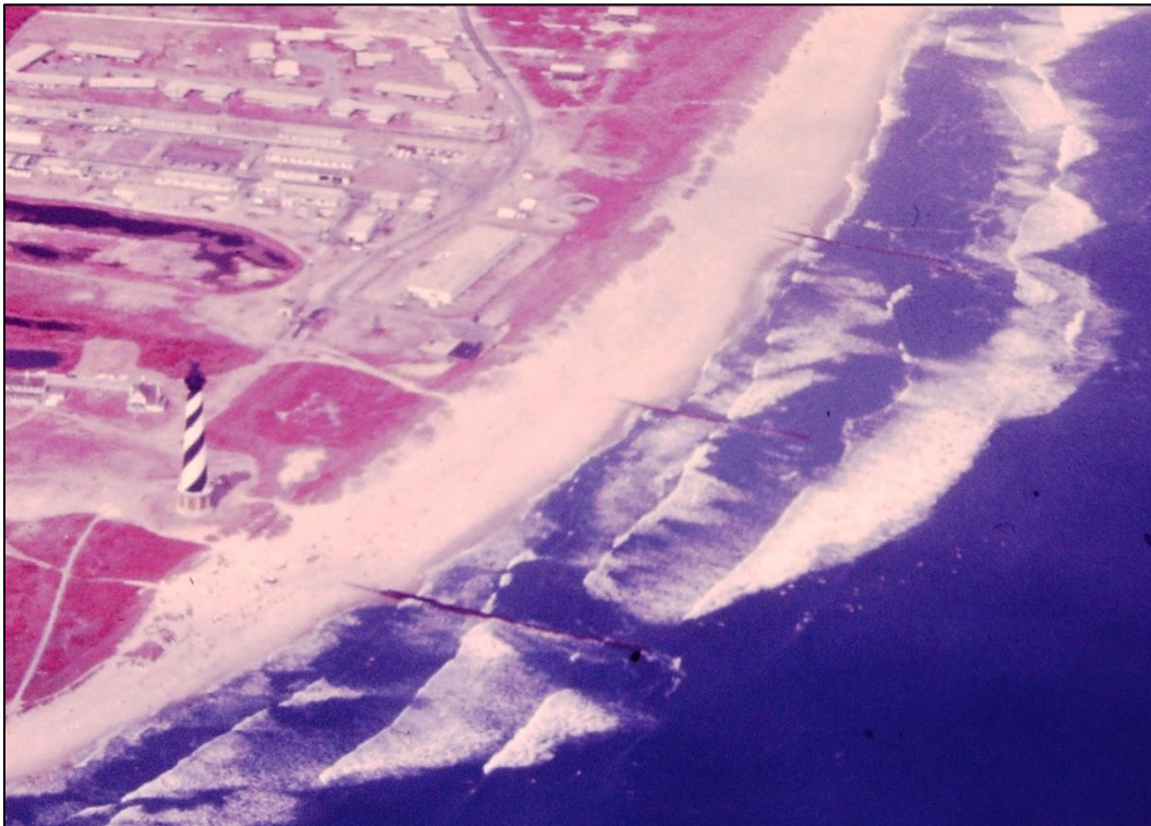
Figure A. Much of the original 1,670 ft length of the three groins remained in place as of September 1978 as shown here. Photo by T. Kana.
