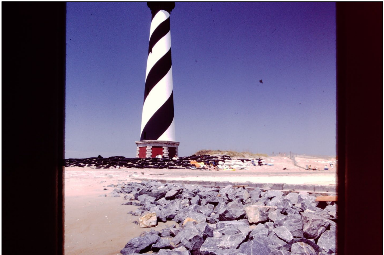
Figure B. By 1984, following the landward extension of the southernmost groin by 300 ft, armor stone scour protection had been installed along the structure and sandbags had been installed at the lighthouse. Photo by T. Kana.
