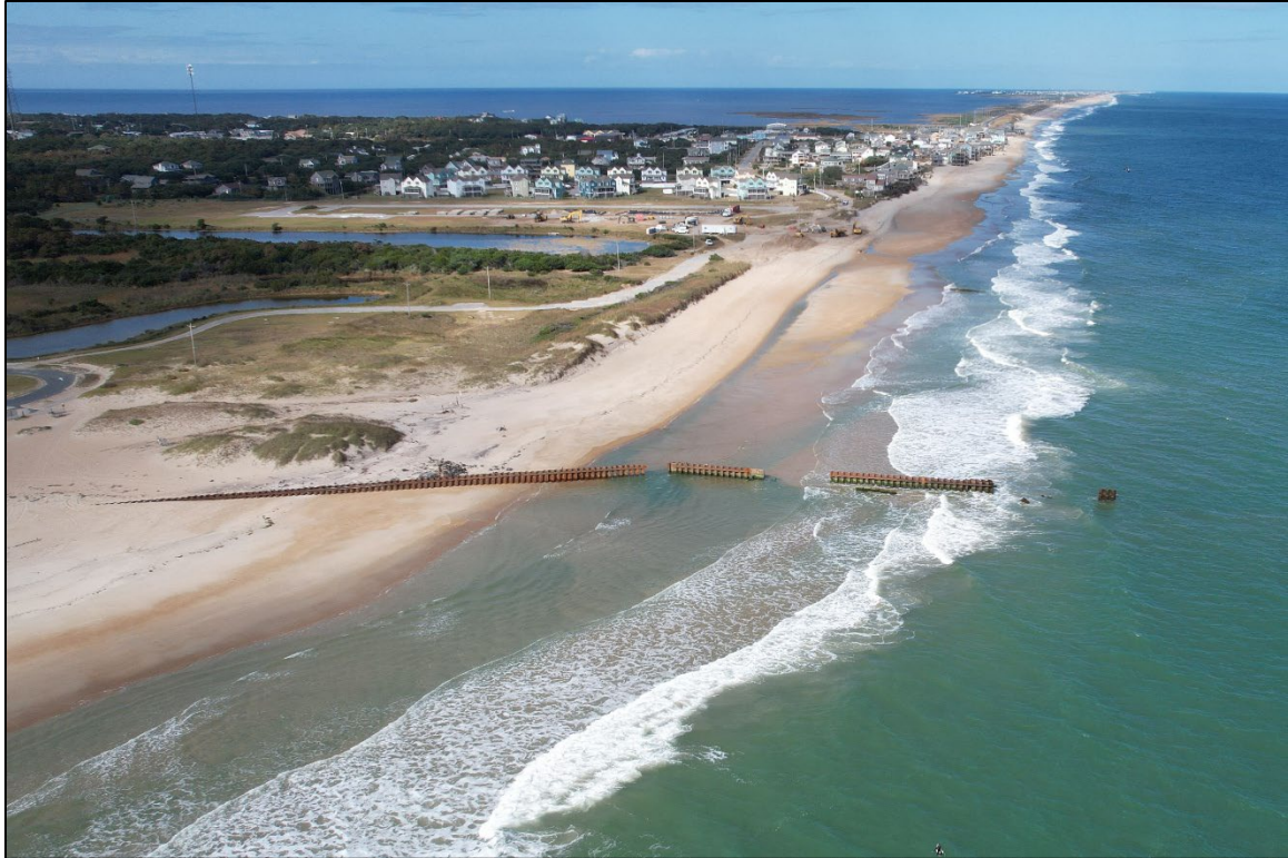
Figure D. As of late 2024, approximately 410 ft of the sheet piles remain in place along the original linear footprint of the southernmost groin. Photo by D Giles.
