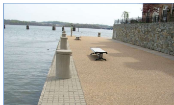
Windmill Hill Bulkhead, Alexandria, VA
