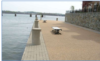
Windmill Hill Bulkhead, Alexandria, VA
