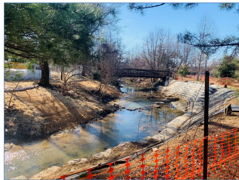
Emergency stream bank repair, DC
