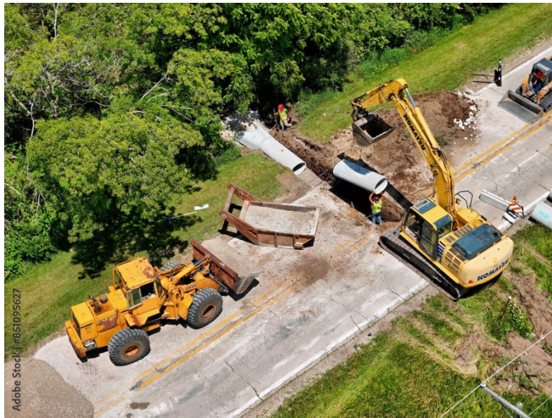
Culvert Construction
