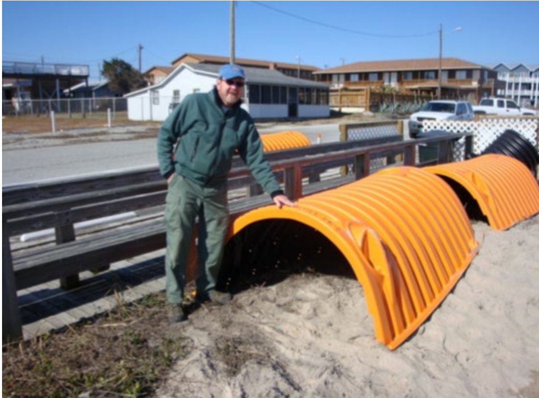
Dune Infiltration System at Kure Beach
