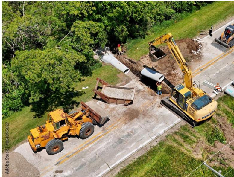
Culvert Construction
