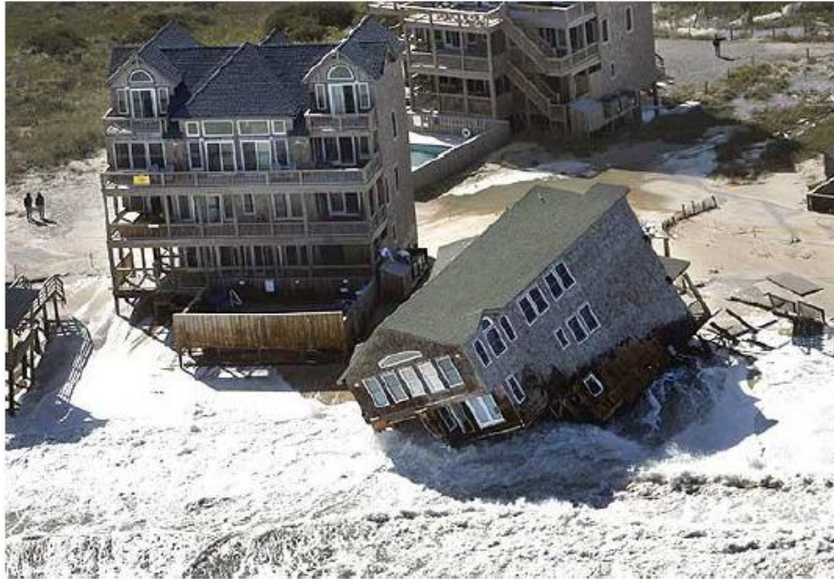
Figure 4. Collapsed exception house in 2008, 4 years after construction.
