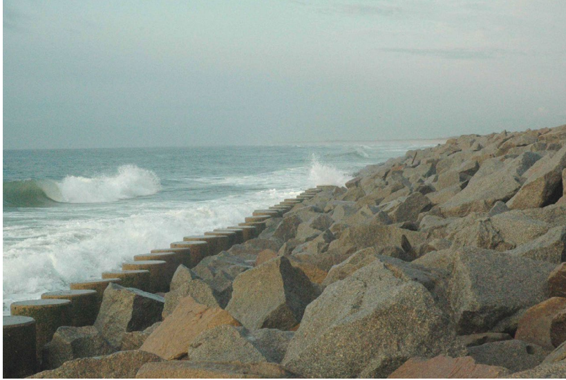
Figure 4. South end of the Fort Fisher revetment.
