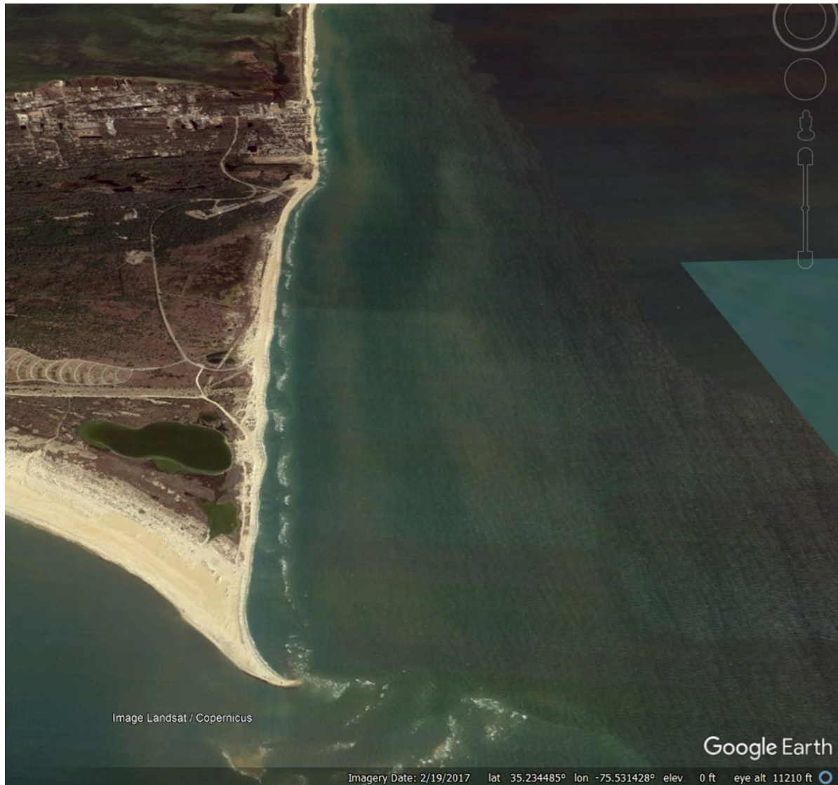
Figure 6. Oblique view of Buxton groins looking north from Cape Hatteras in 2017. When functional the groins have slowed the rate of erosion farther north with the tradeoff of creating a sand deficit farther south.
