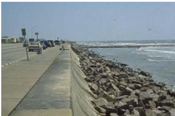
Figure 13. The Galveston Seawall.
