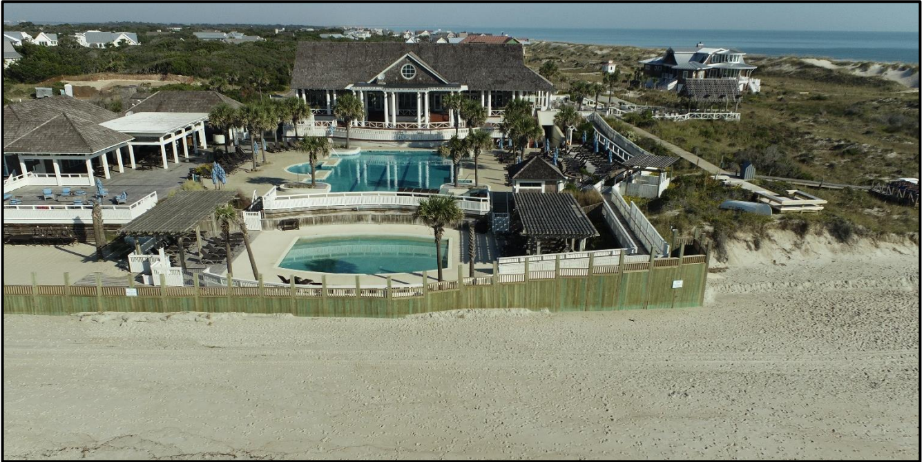
Figure 10: Drone imagery from November 8, 2023, approximately 1.5 years post-installation of the sandbags. Potential settling of the sandbags and an accretional event resulted in temporary covering of the sandbags. Image courtesy of Olsen Associates, Inc.
