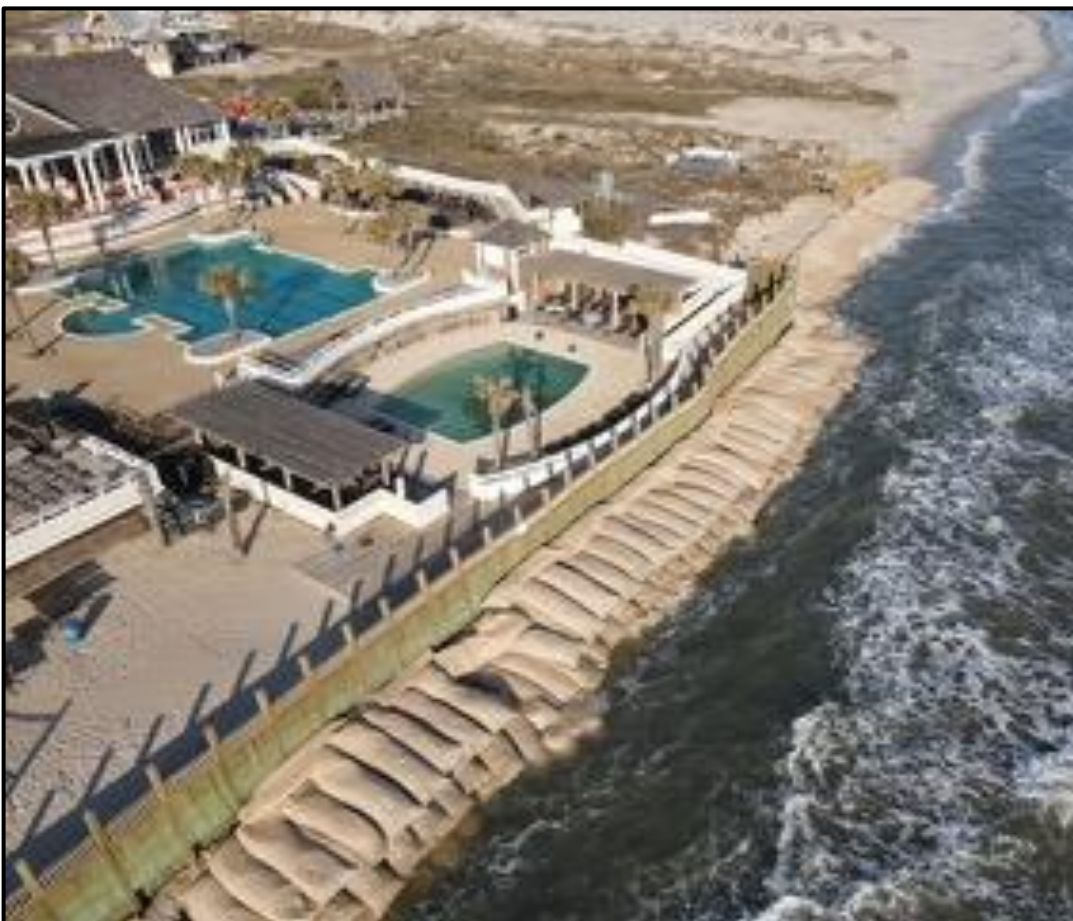
Figure 7: March 2023 drone imagery of a high-water event impacting the sandbags approximately 10-months post-installation. Image courtesy of the Shoals Club.
