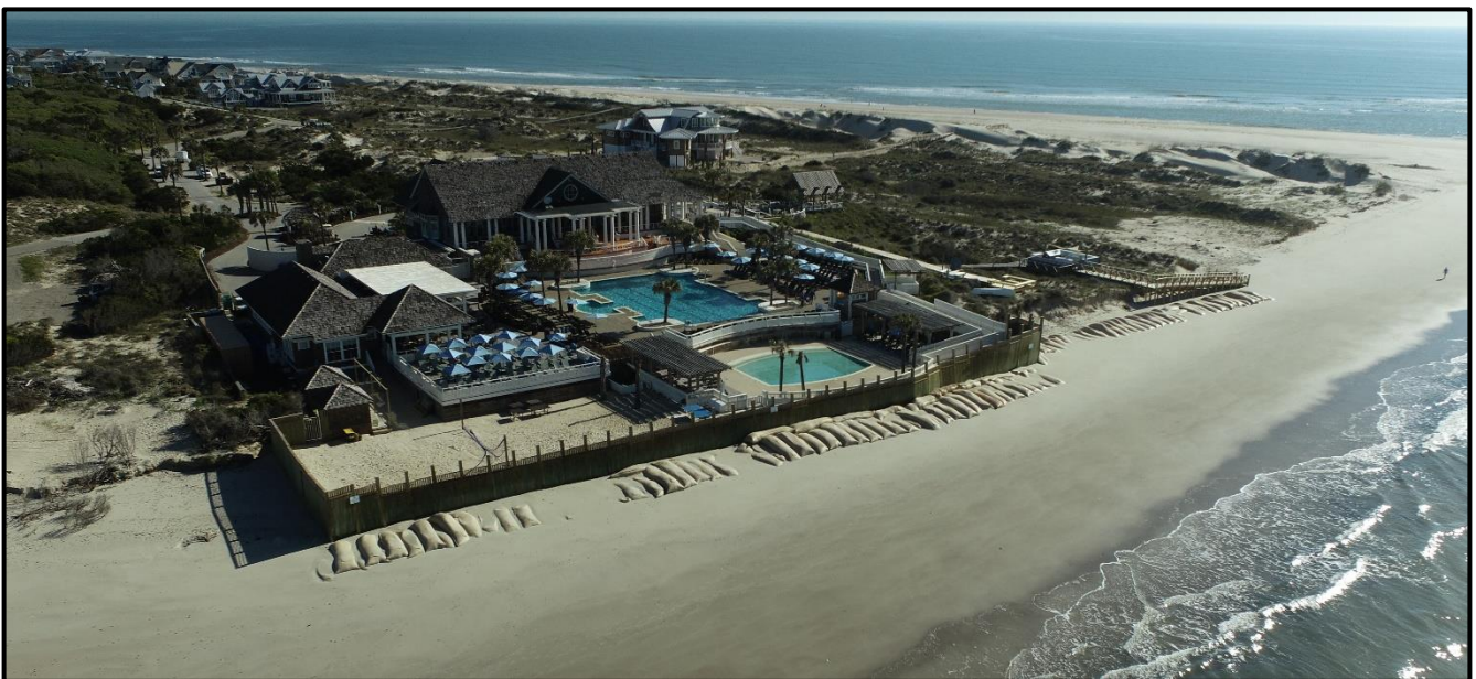
Figure 9: Drone imagery from April 13, 2023, approximately 11-months post-installation of the sandbags. Image courtesy of Olsen Associates, Inc.
