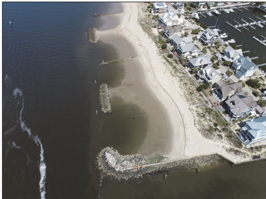
Figure 3.12: Northward looking view of the Row-Boat-Row shoreline detached breakwaters. (April 2024 Photo).
