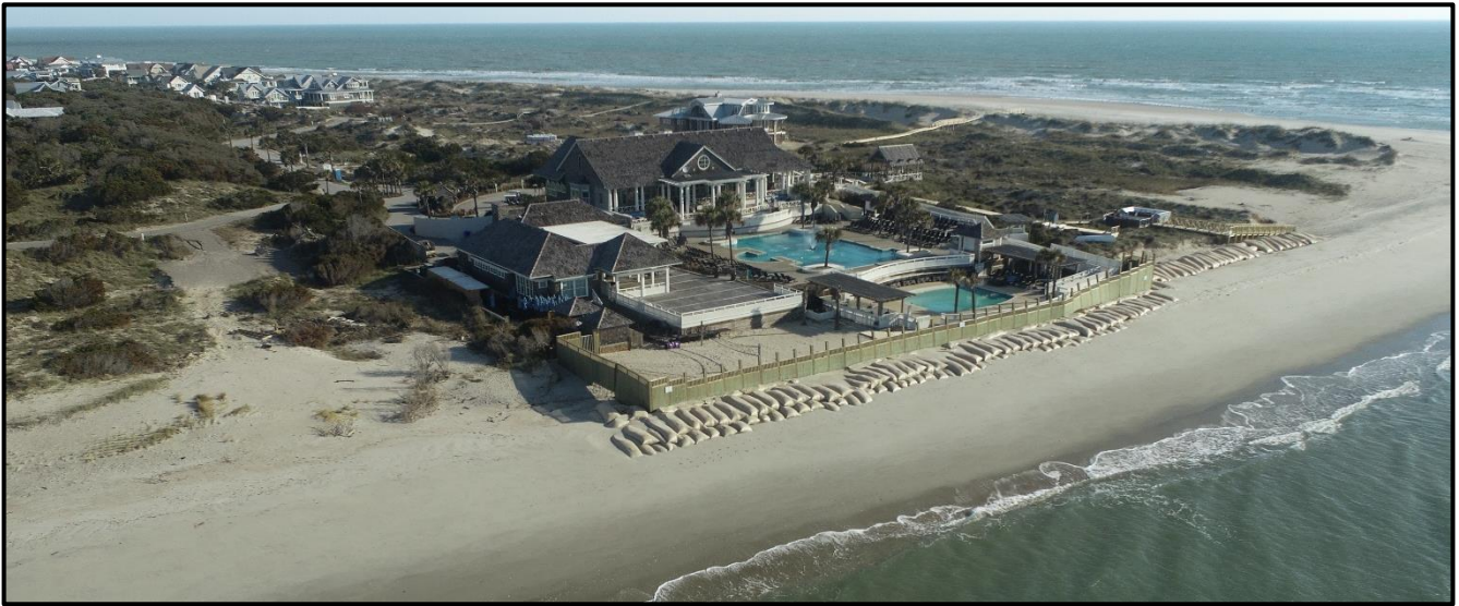
Figure 6: Drone imagery from November 1, 2022, 6-months post-installation of the sandbags. Note the height of the bags relative to the top of the wooden fence. Image courtesy of Olsen Associates, Inc.
