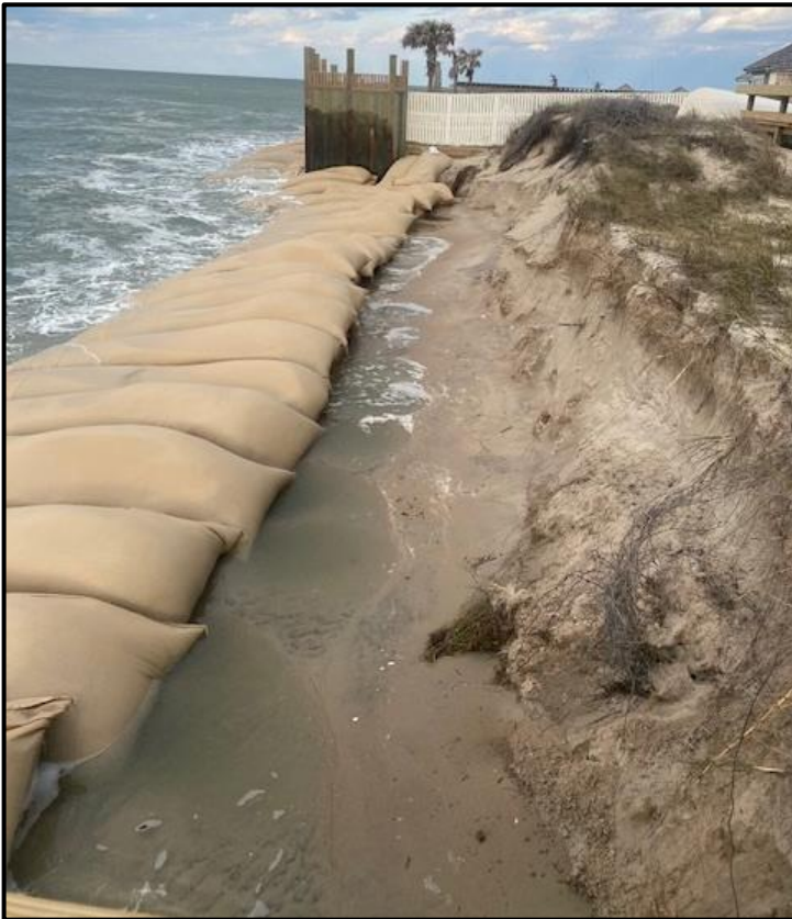
Figure 8: March 2023 imagery of a high-water event impacting the sandbags approximately 10-months post-installation. Image courtesy of the Shoals Club.
