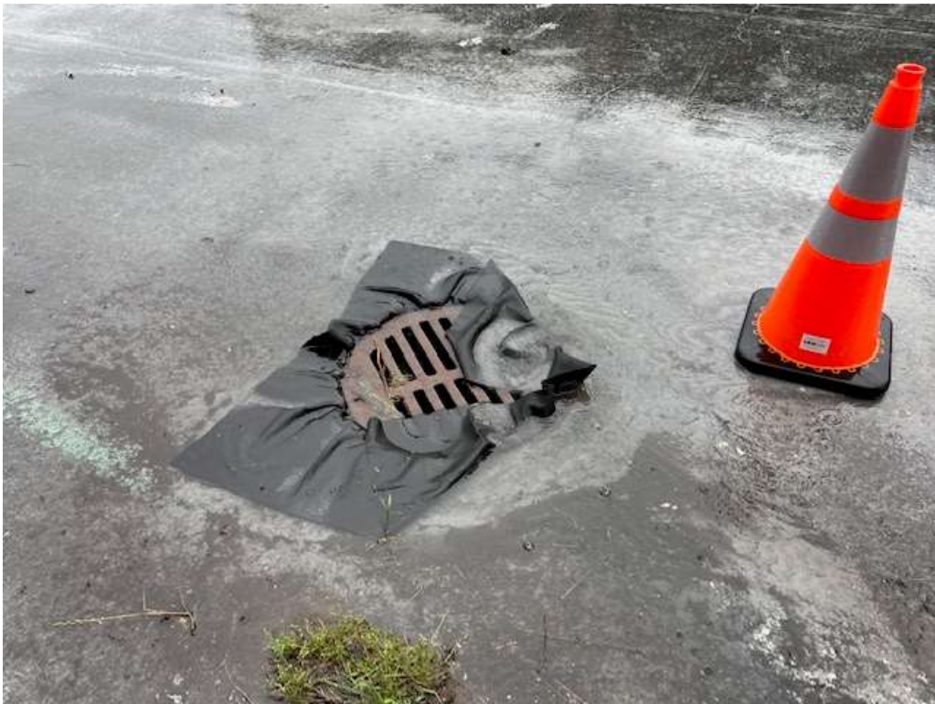
Silt sacks installed in yard inlets.
