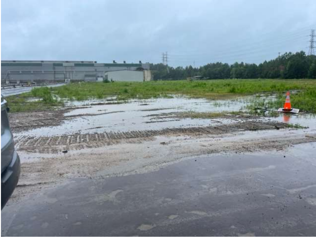
Exposed sediment from hauling traffic.
