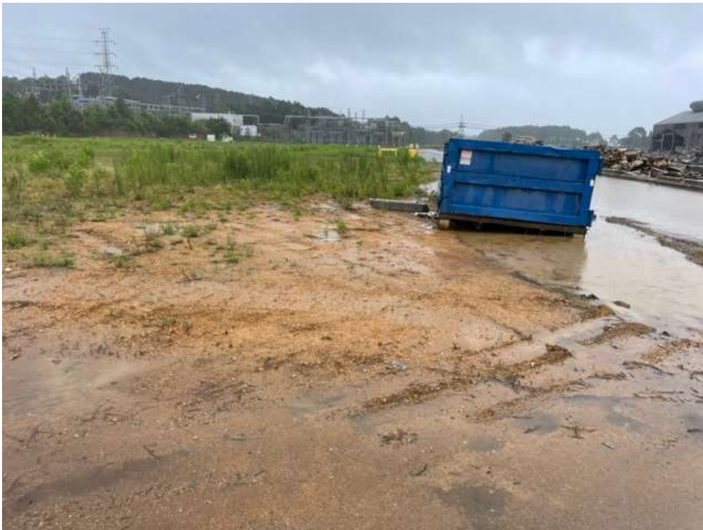
Exposed sediment from hauling traffic.
