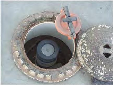
Dual point vapor recovery involves a separate pipe to the tank, located in its own sump.
