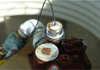
An Automatic Line Leak Detector (ALLD), either mechanical or electrical, detects catastrophic leaks of 3.0 gph or more.
