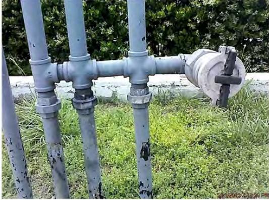
Dual point vapor recovery may be manifolded so the vapor from all the tanks is recovered from one port.
