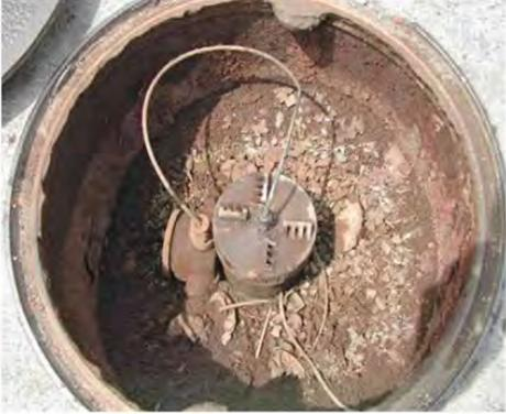
If you are using an Automatic Tank Gauge (ATG) for your tank leak detection, the inspector will check the ATG port to make sure that the tank probe is capped and all the wires are intact. This is a picture of an open ATG port with the top of the ATG cap visible.
