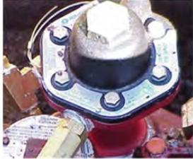
**Electronic Line Leak Detectors (ELLD)**
