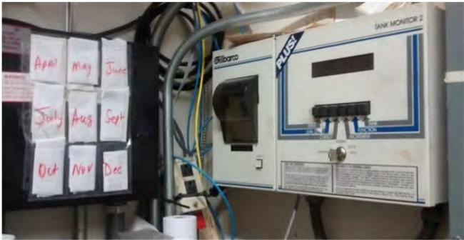
A photograph showing an Automatic Tank Gauge (ATG) unit, labeled "TANK MONITOR 2" and "PMS", installed in a control room. To the left of the unit is a calendar with months from April to December written on it. The ATG unit has a digital display and various control buttons.
