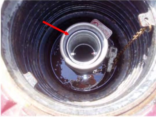
Coaxial vapor recovery is a part of the fill port inside the spill bucket. Note the double ring.
