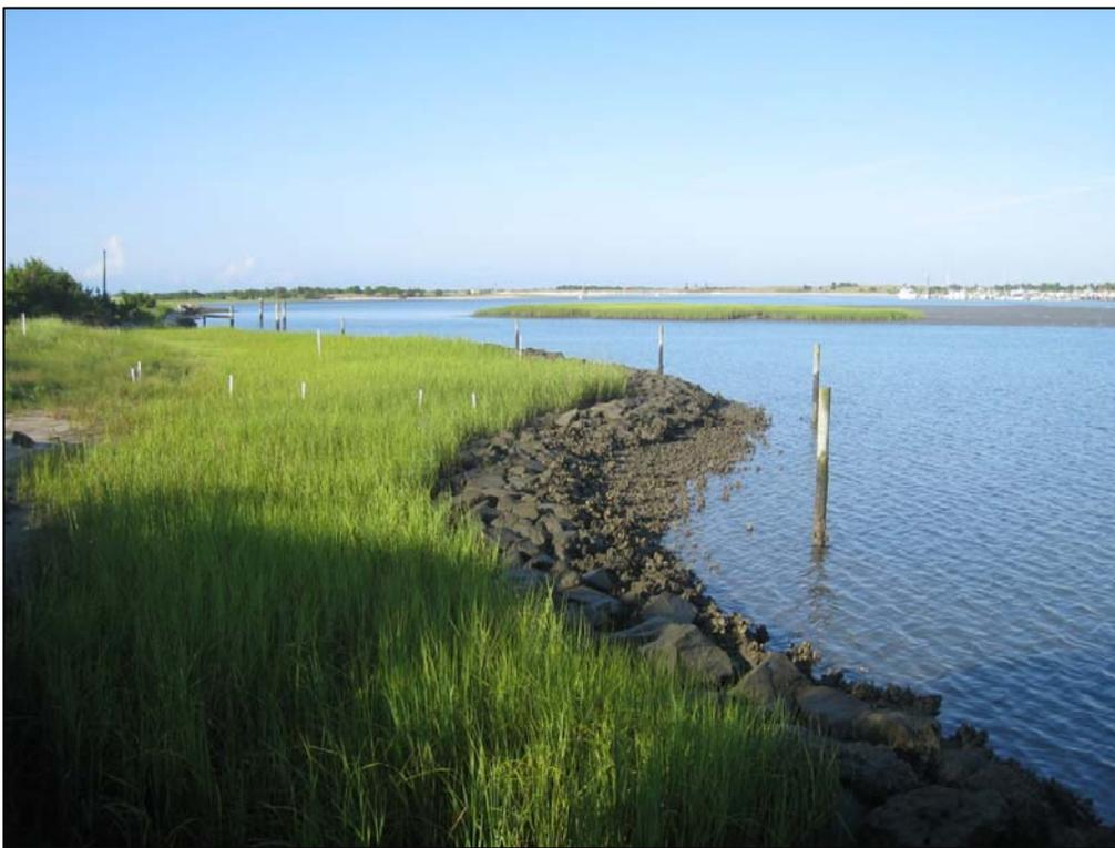
**Figure 1.** Riprap Marsh Sill at Pivers Island, NC.
