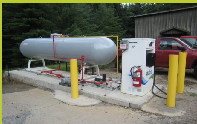
The 6.8L, V-10 Starcraft Allstar 25 shuttle bus (shown above) now runs primarily on propane and can fill up from the on-site Alliance AutoGas tank (shown below) near the security building.
