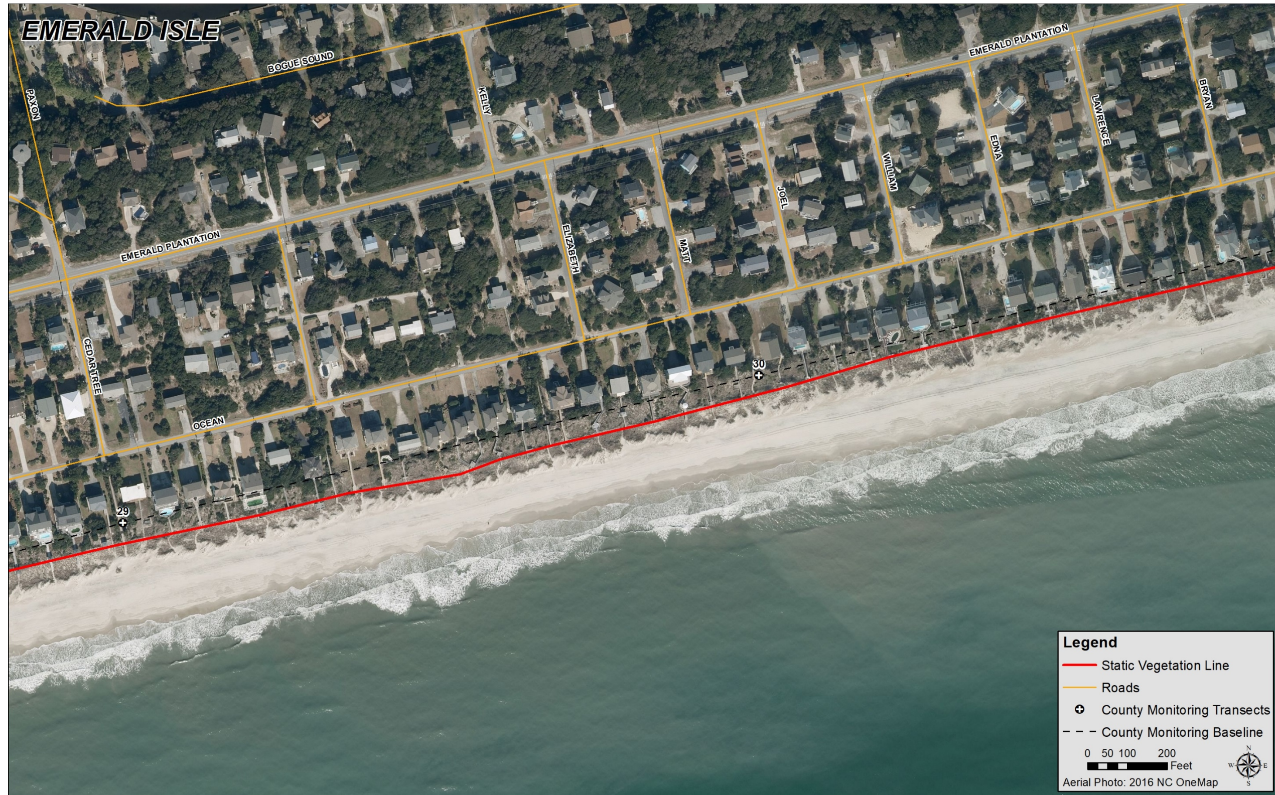
Figure 2-5. Eastern Emerald Isle Static Vegetation Line (3 of 10)
