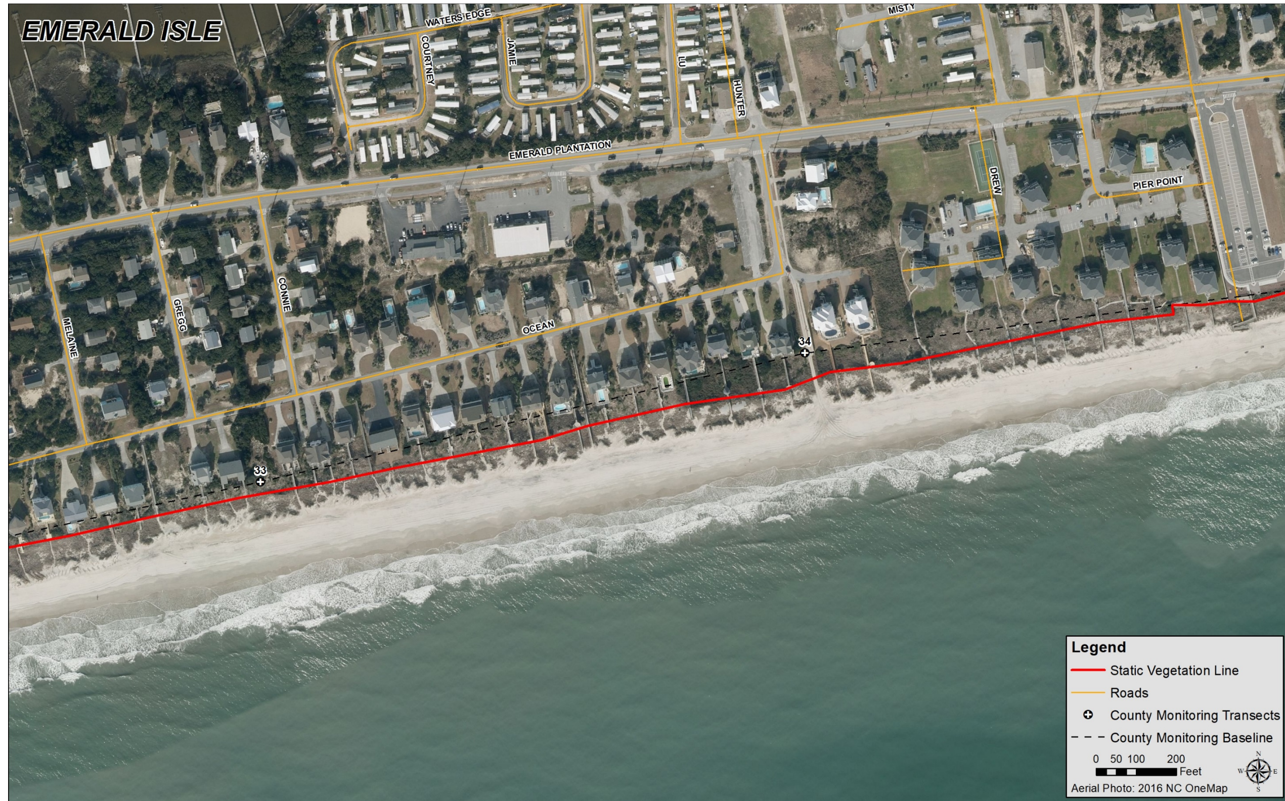
Figure 2-7. Eastern Emerald Isle Static Vegetation Line (5 of 10)
