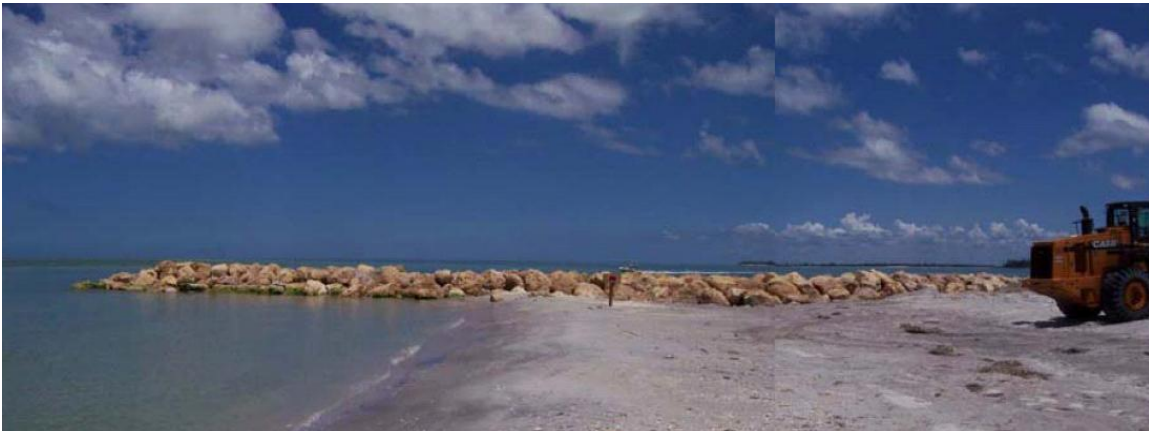
Figure IV-7. 2006 Terminal Groin at Captiva Island
