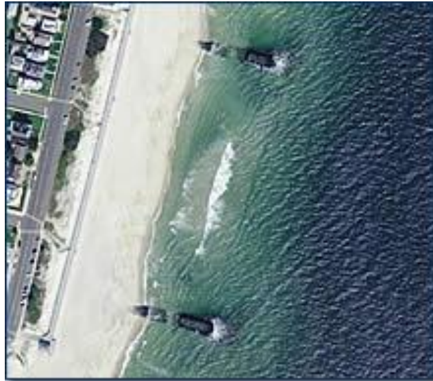
Figure IV-25 Example of Notched Groins (New Jersey DEP Website)
