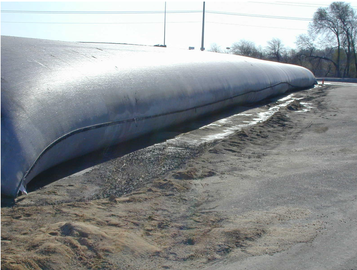
Figure IV-24. Example of a Geotextile Tube
