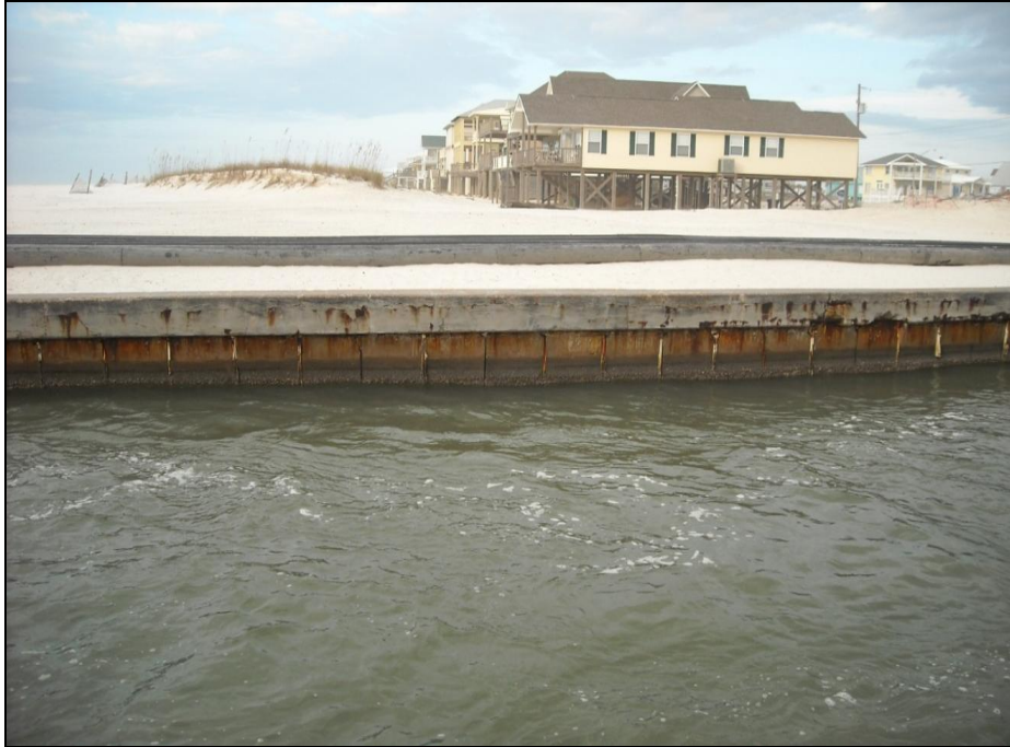
Figure IV-20. Example of Concrete Sheet Piles
