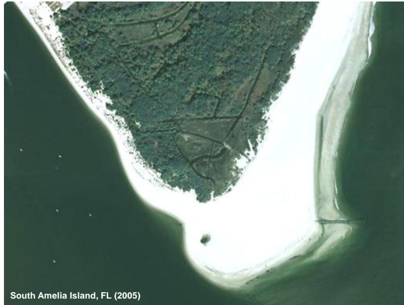
Figure II-40. Amelia Island Terminal Groin
