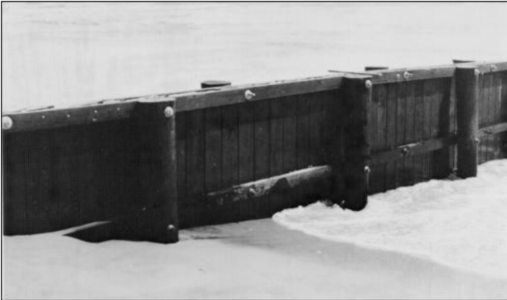
Figure VI-6. Example of a Timber Groin
