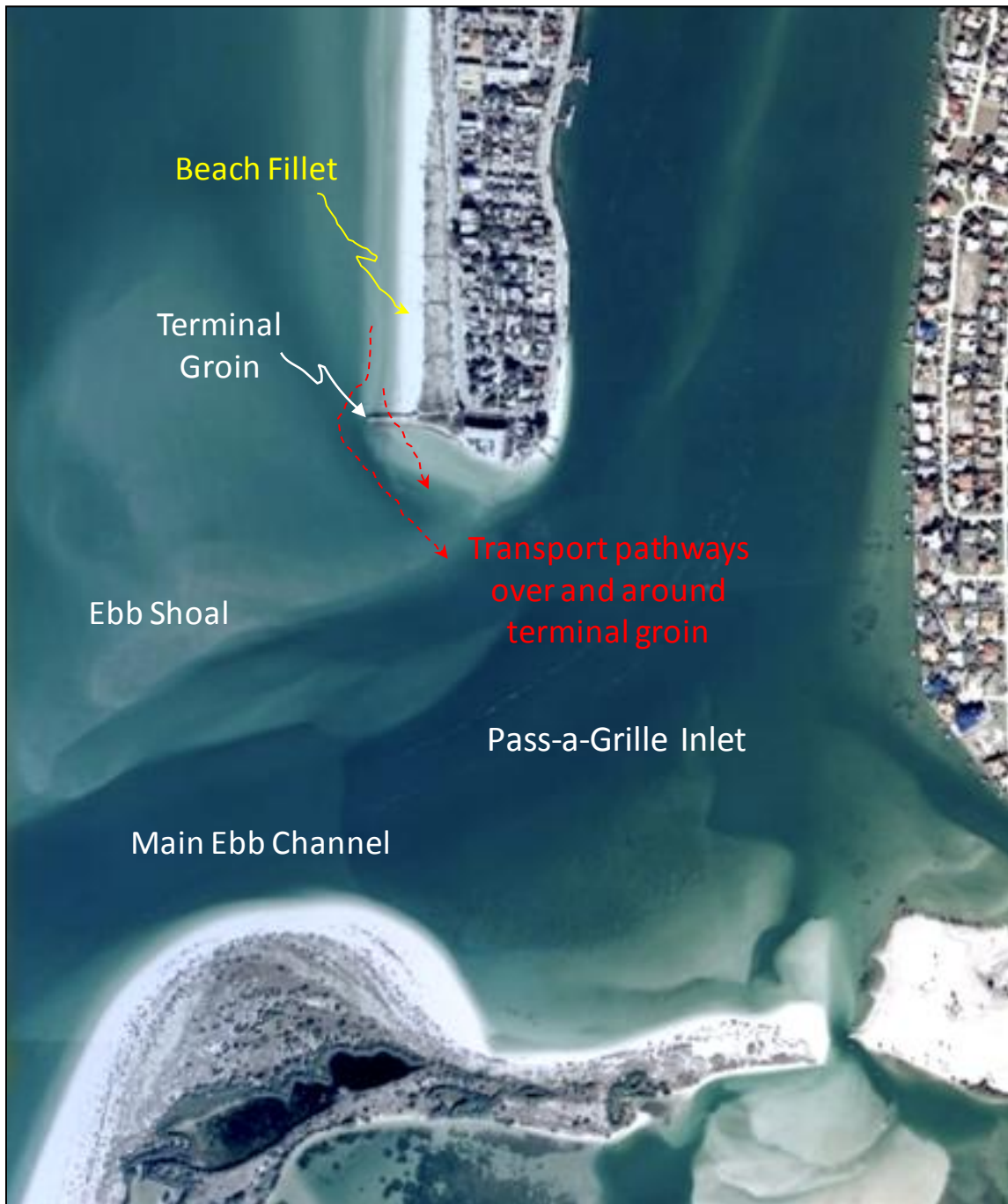
Figure II-1. Terminal Groin at Saint Pete Beach, Florida
