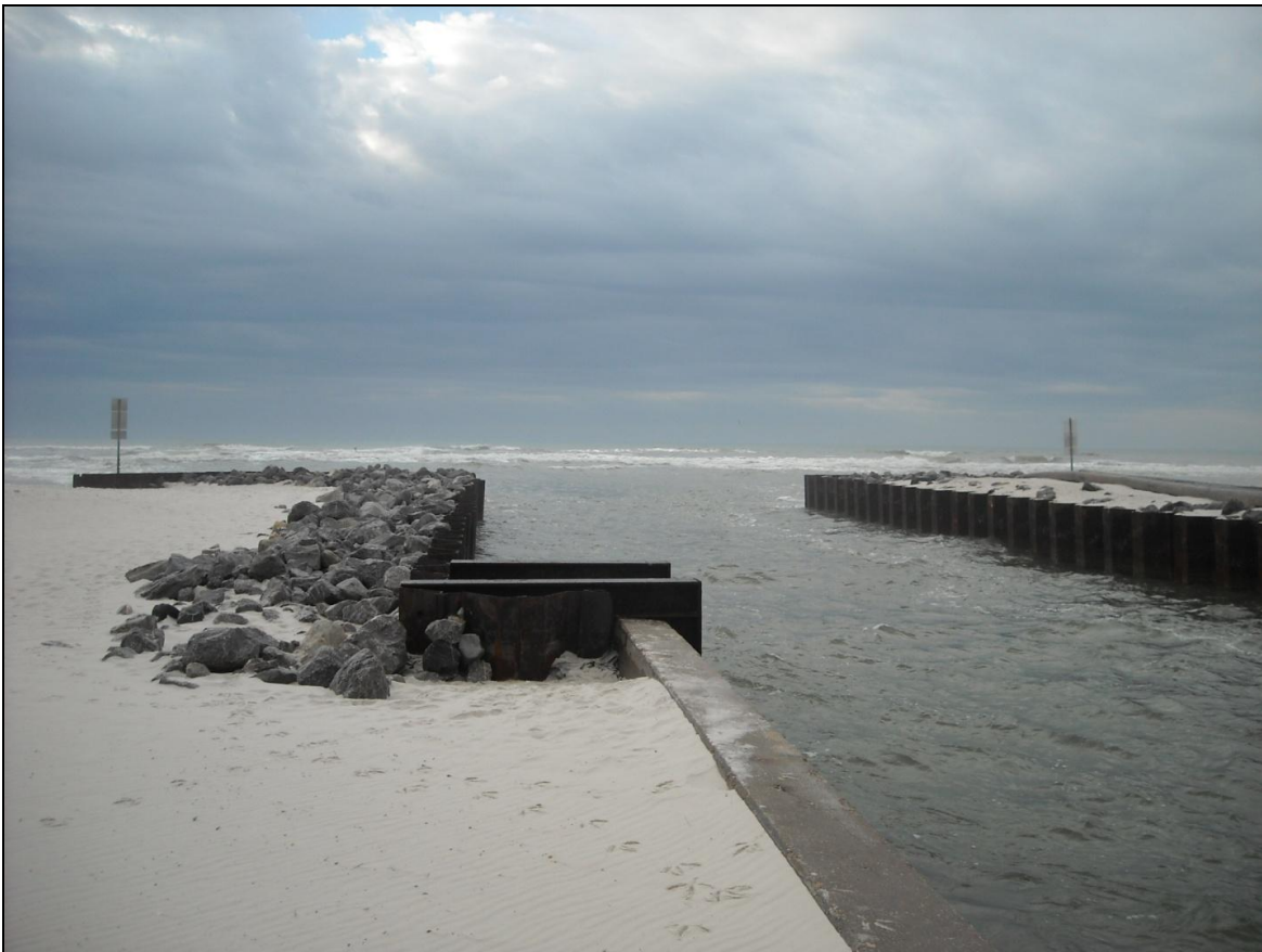
Figure IV-22. Example of Steel Sheet Pile Terminal Groin
