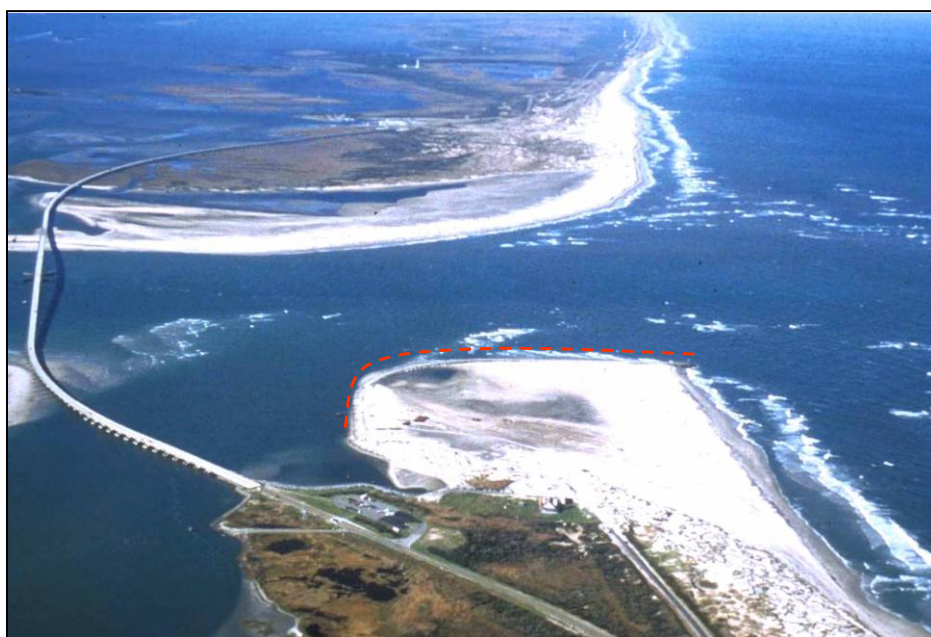
Figure II-6. Oregon Inlet Terminal Groin & Revetment
