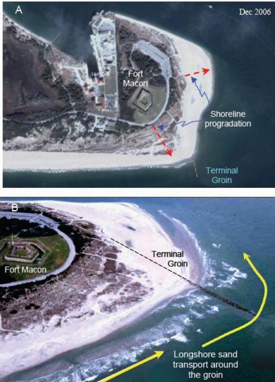
Figure II-27. Photographs Illustrating Progradation of the Beach West of the Groin and Along Inlet Shore. Dashed line indicates extent of groin beneath the beach
