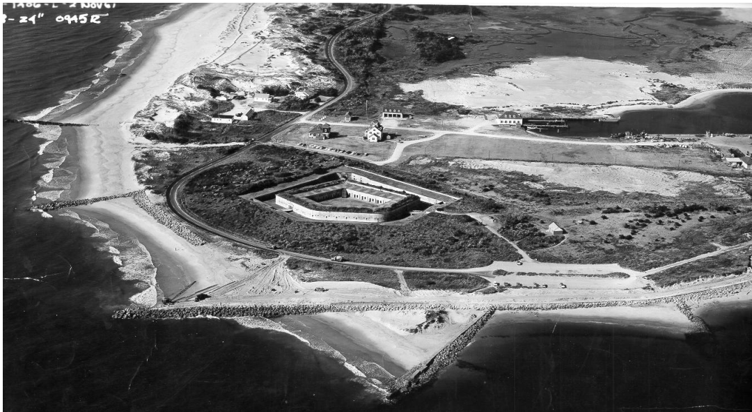
Figure II-24. Fort Macon Revetment-Groin Protection (1961)
