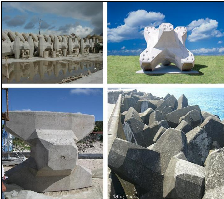
Figure IV-21. Examples of Concrete Armor Units
