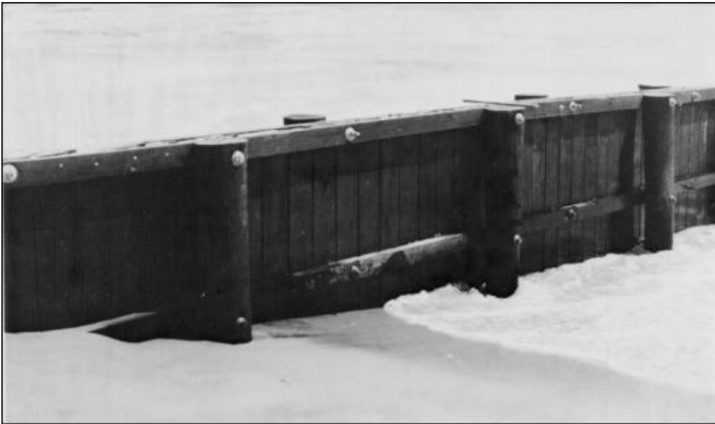
Figure IV-23. Example of a Timber Groin
