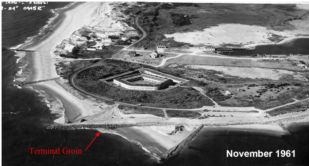
Figure IV-4. Fort Macon Terminal Groin Initial Construction (1961)
