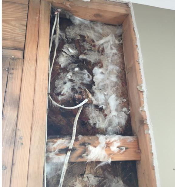
Water damage around French doors on lowest two levels.
