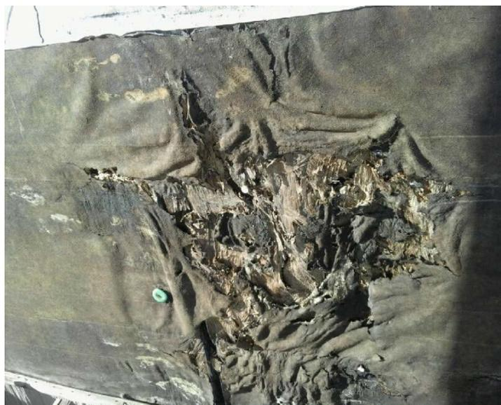
Water damage rotted away house boards. Interior o bedroom and bath on lowest living level (2<sup>nd</sup> story)
