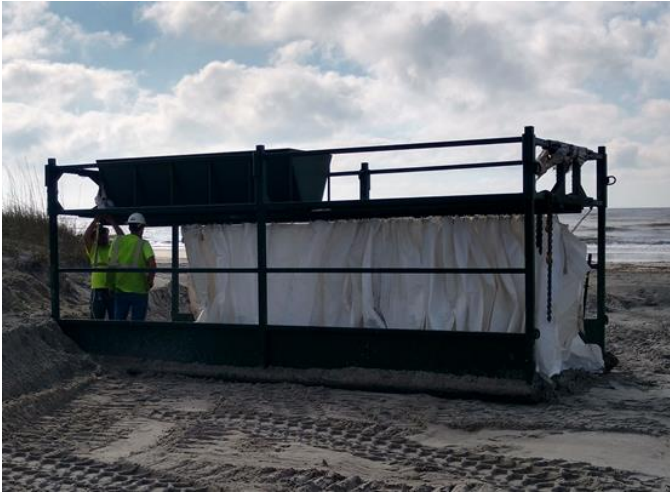
Illustration I: Installation Platform for concrete for quick and efficient fill.
