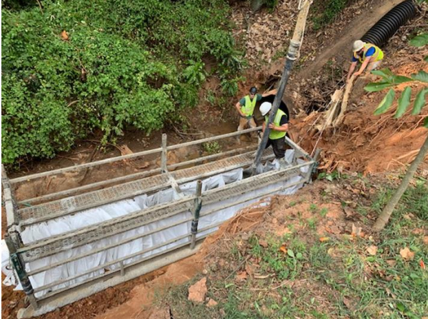
Illustration I: Installation Platform for concrete for quick and efficient fill.
