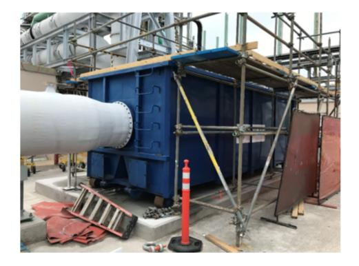
DAQ required Chemours to install carbon adsorbers in May of 2018. The carbon adsorber units are expected to reduce the overall GenX air emissions by 40%.
