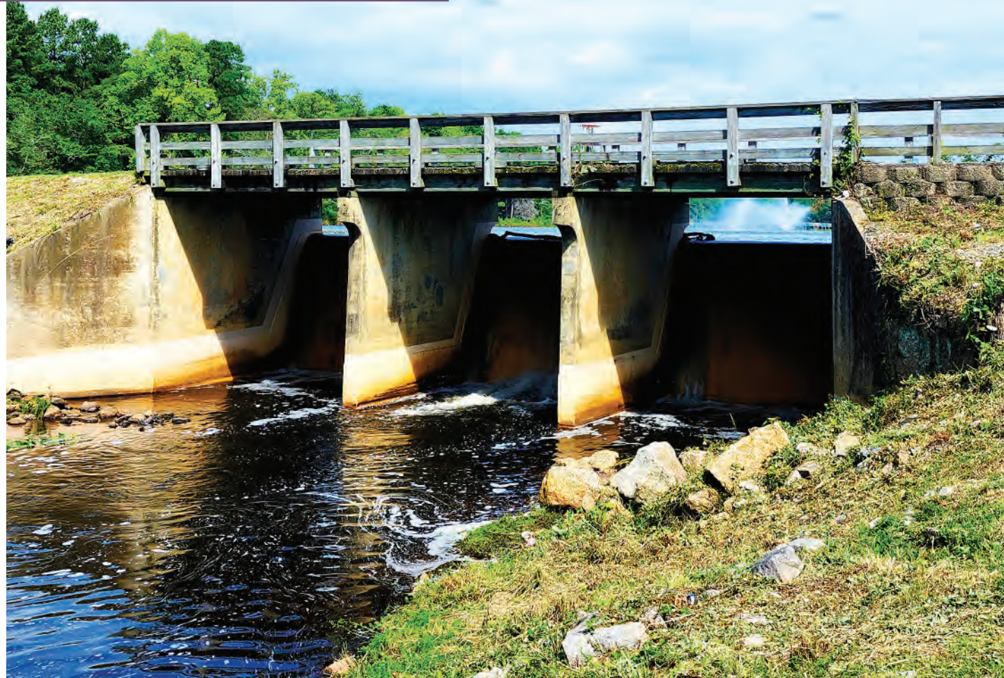
Bridge in Aberdeen Lake Park, North Carolina, USA
