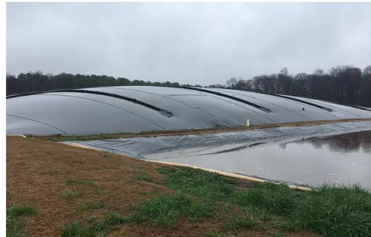
Methane accumulates under a cover at a hog waste lagoon (anaerobic digestion).
