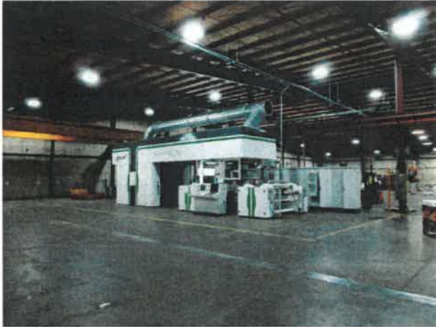
Picture 1: Overall view of the new press under construction in the printing facility.
