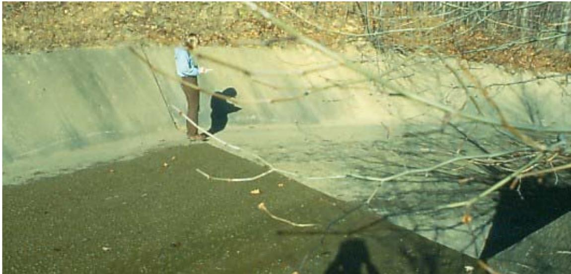
Flow entering the joint of a spillway floor slab.
