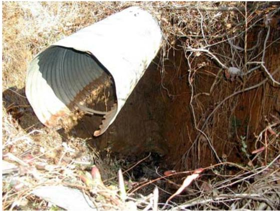
Right: Corroded pipe spillway.
