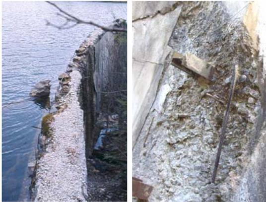
Right: Spalling Concrete.
