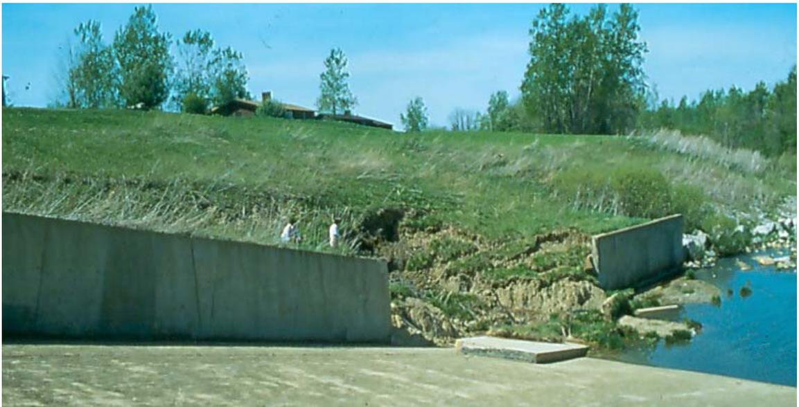
Collapse of spillway wall section.
