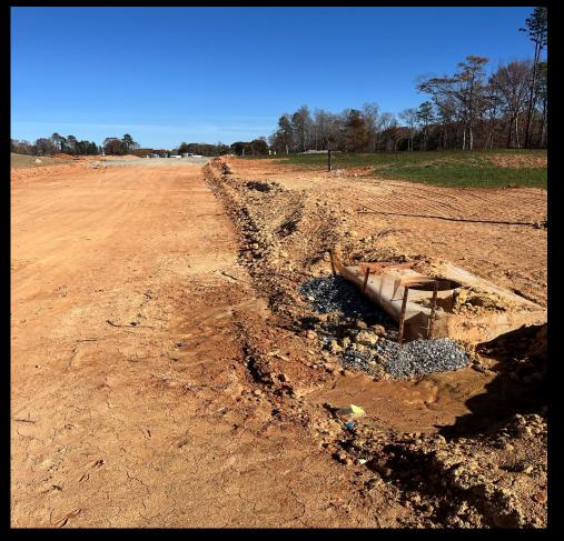
Add floc logs to storm drain system for passive treatment in every rain event
