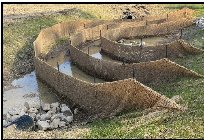
Figure 6.65c , Example of porous baffles installed in skimmer basins
