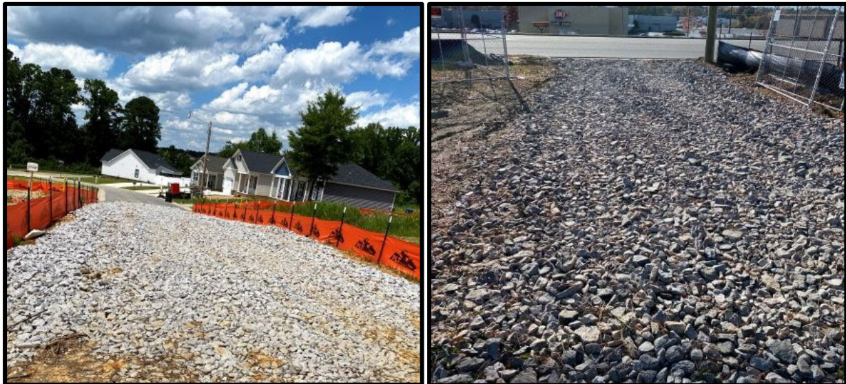
Figure 6.06b, Stone Entrance/Exit keeps sediment from leaving the construction site
