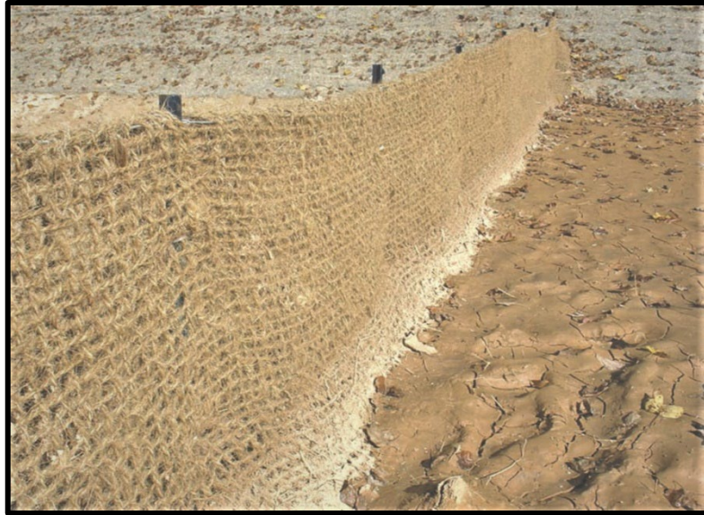
Figure 6.65d , Close-up of a porous baffle made of 700 g/m 2 coir erosion blanket
