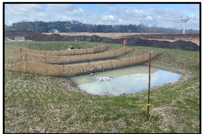
Figure 6.65c , Example of porous baffles installed in skimmer basins
