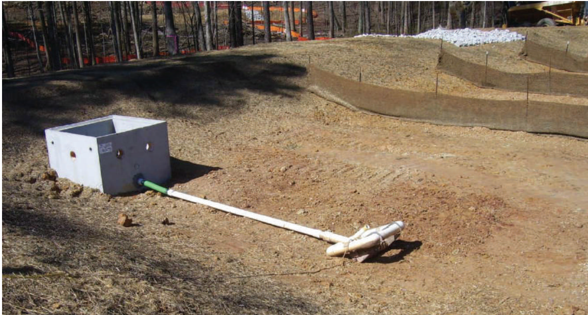
Figure 6.61b Sediment basin with skimmer attached to riser for dewatering. Photo Credit: Town of Apex
