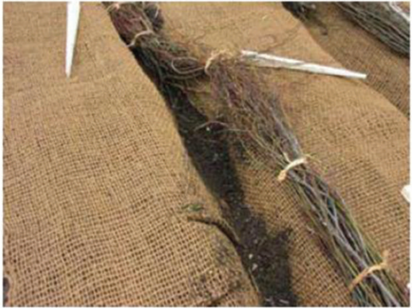
Figure 6.72c Combining fascines and fabric
