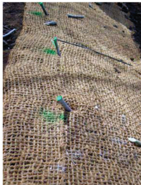
Figure 6.72d Live cuttings installed in fabric
