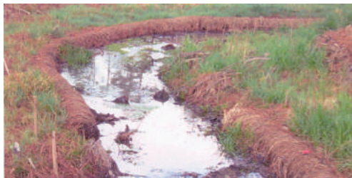
Figure 6.72b Coir log installation, NC Ecosystem Enhancement Program
