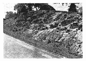
FIGURE 3.—Jointed and partially weathered granite near Woodleaf, Rowan County. Although typical of many massive granites, the rock is not as completely decomposed as most other rocks.
