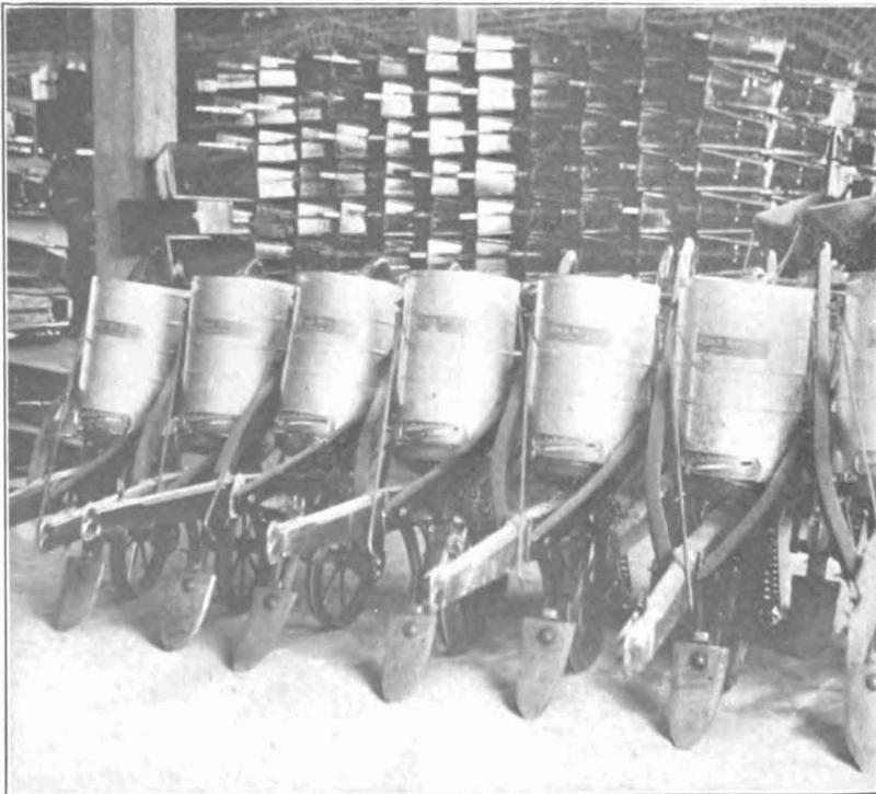
B. Interior of a North Carolina agricultural implement factory. Oak is the only wood used in the manufacture of the small fertilizer distributors shown in this plate, the wood being employed for plow beams and handles.
