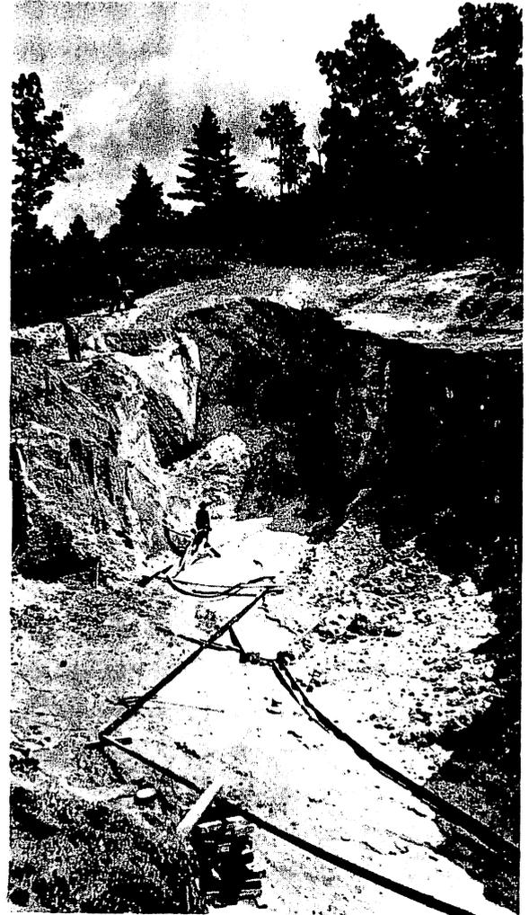
Figure 15. Veins in the South Mountain belt were commonly worked by hydraulicking methods, such as the operation shown here.
