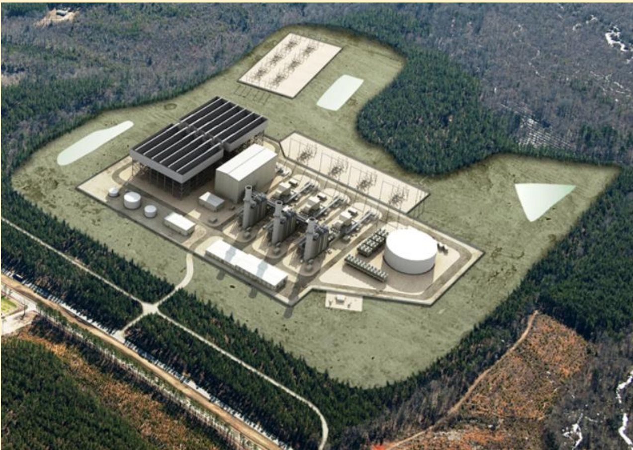
Brunswick County Power Station, Virginia – see URL http://www.power-technology.com/projects/brunswick-county-power-station-virginia/ .
