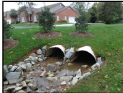
Stormwater pipes transfer water from the street directly into streams.
