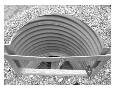
The traditional riser barrel has been replaced with a flashboard riser that allows the researchers to retain water in the riser and pool. A PAM floc log is suspended in the barrel. McLaughlin says this is the ideal place to use a floc log.
