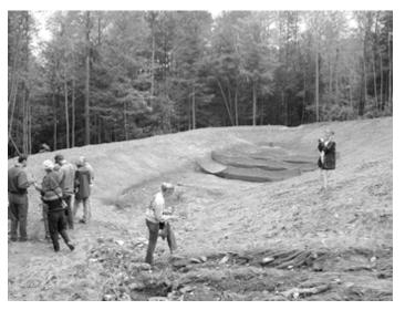
Jute baffles in this large riser-barrel basin have slowed water velocity and encouraged sediment to drop out in forebays just below the inlet. One side of the first baffle has collapsed. McLaughlin recommends using tree protection fence as the first baffle because it can better withstand the force of water rushing into the basin.
