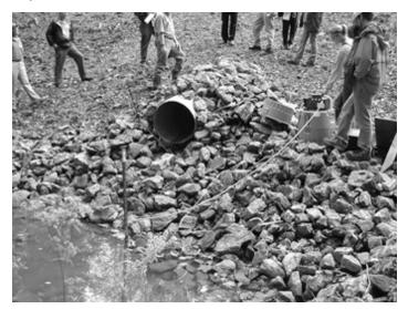
A PAM floc log is secured just below the basin outlet pipe where flow will dissolve more PAM and encourage flocculation in this settling pool, which is at the end of the PAM-BMP train. Sampling here has shown turbidity as low as 50 NTU.
